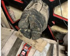
Next, all the internal bearing support metalwork and associated wedges holding the wheel to the shaft had to be removed. Not as easy as it looked! Here the shaft is supported by a trolley jack whilst wedges are removed.
