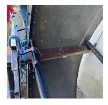
At the same time as removing the outside bearing we had to prevent the wheel from rolling forward. To do this we fixed a wooden brace across the spokes. This was then tied to the steel lifting stanchion above. This stanchion is mounted in the mill wall above the water wheel.
